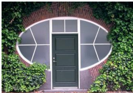
98 Kloakpumpestation, Gl. Lundtoftevej
